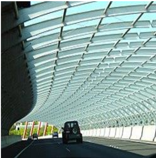
Figure 3: The sound tube in Melbourne, Australia is designed to reduce roadway noise without detracting from the area's aesthetics.
